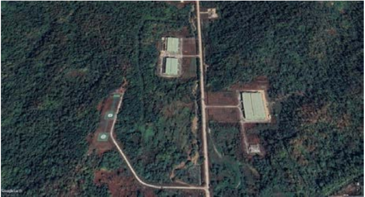
Helipads visible at KaPaSa 24
